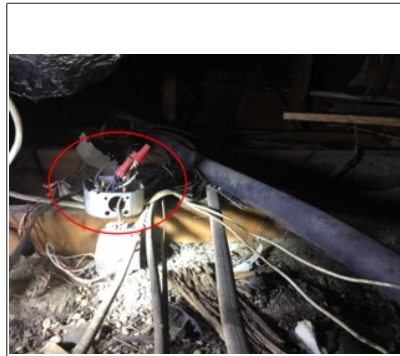
Garage attic access
