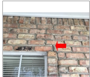
Front exterior window right side of entrance
