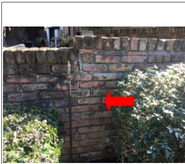
Front left exterior retaining wall separation.
