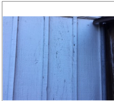
Left side rear exterior wall
